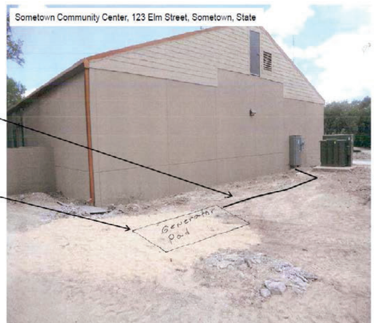
Figure 4. Ground-level photograph showing proposed ground disturbance area.
