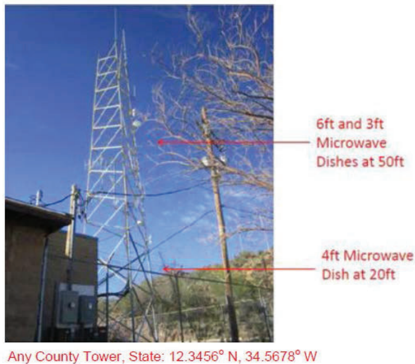
Figure 5. Ground-level photograph showing proposed locations of new communications equipment on an existing tower.
