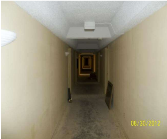
Photograph #13 General interior view of the subject building
