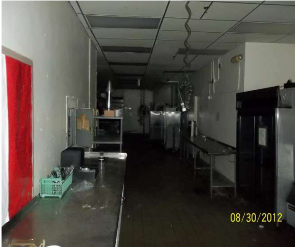
Photograph #3 General interior view of the subject property
