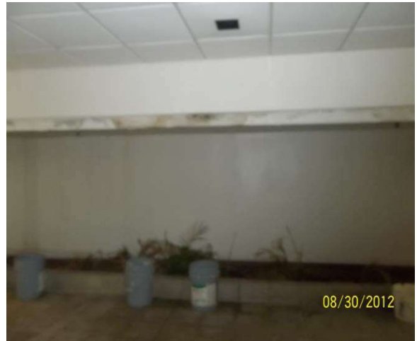
Photograph #10 General Interior view of the subject building
