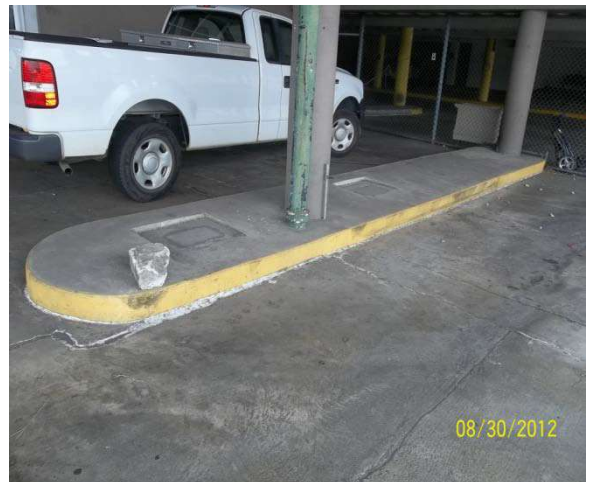
Photograph #16 View of 1 of 2 island dispenser located in the northern portion of the subject site
