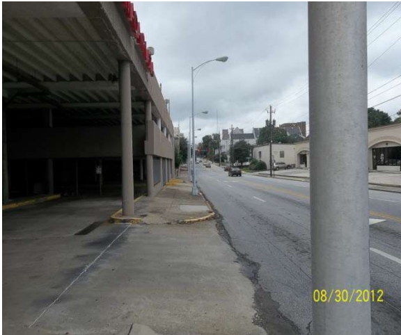
Photograph #19 View from the northern corner of the subject site looking southward along the western property boundary
