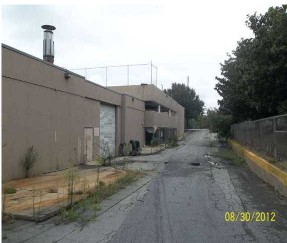
Photograph #29 General exterior view of the back of the subject building
