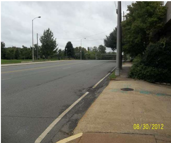
Photograph #21 View from the northern corner of the subject site looking eastward along the northern property boundary
