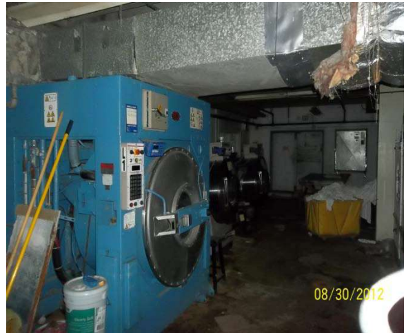
Photograph #8 General interior view of the subject property
