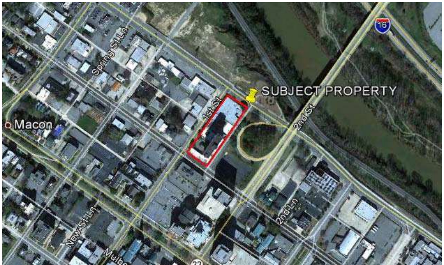
Figure 3 2012 Aerial Photograph Ramada Plaza 108 First Street Macon, Bibb County, Georgia GEC Project #120586.240 Approximate Scale: 1"= 510' Source: Google Earth Website
