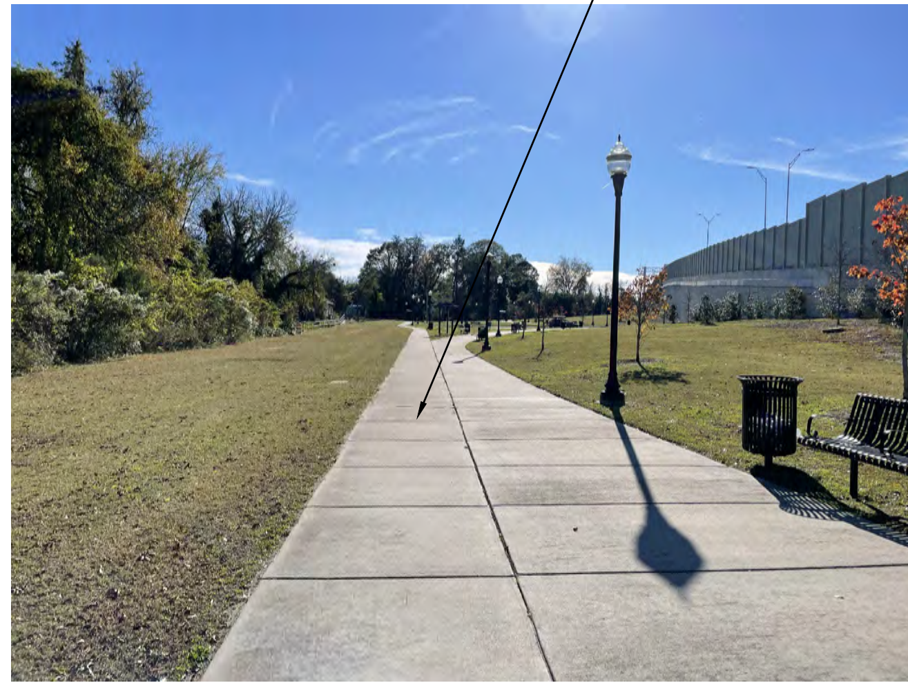
EXISTING CONCRETE WALKWAYS
