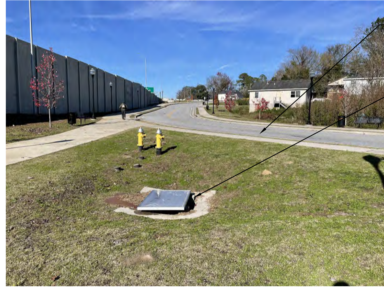
FIFTH AVE WEST EXISTING STORM INLET
