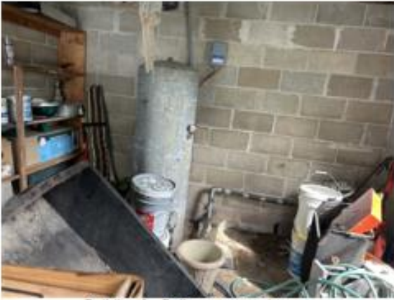
Building 2 - Boiler room, not in use
