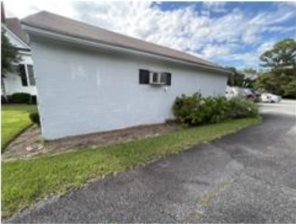
Building 1 back view
