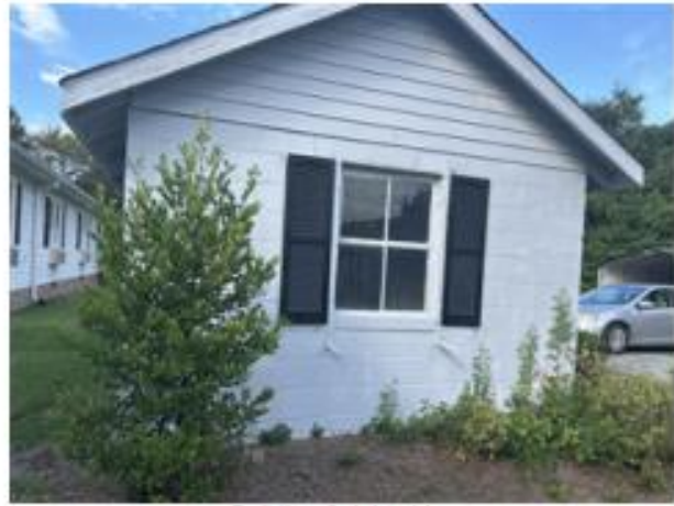
Building 2 right side
