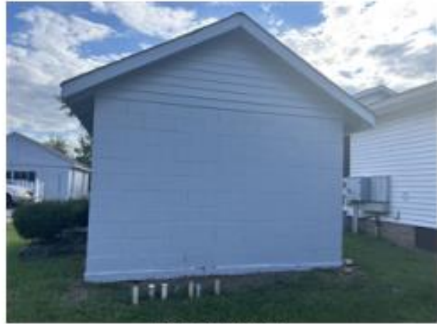
Building 2 left view
